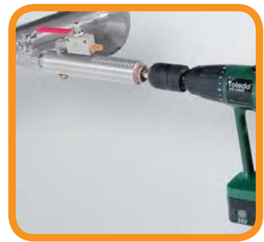
Drilling under pressure
